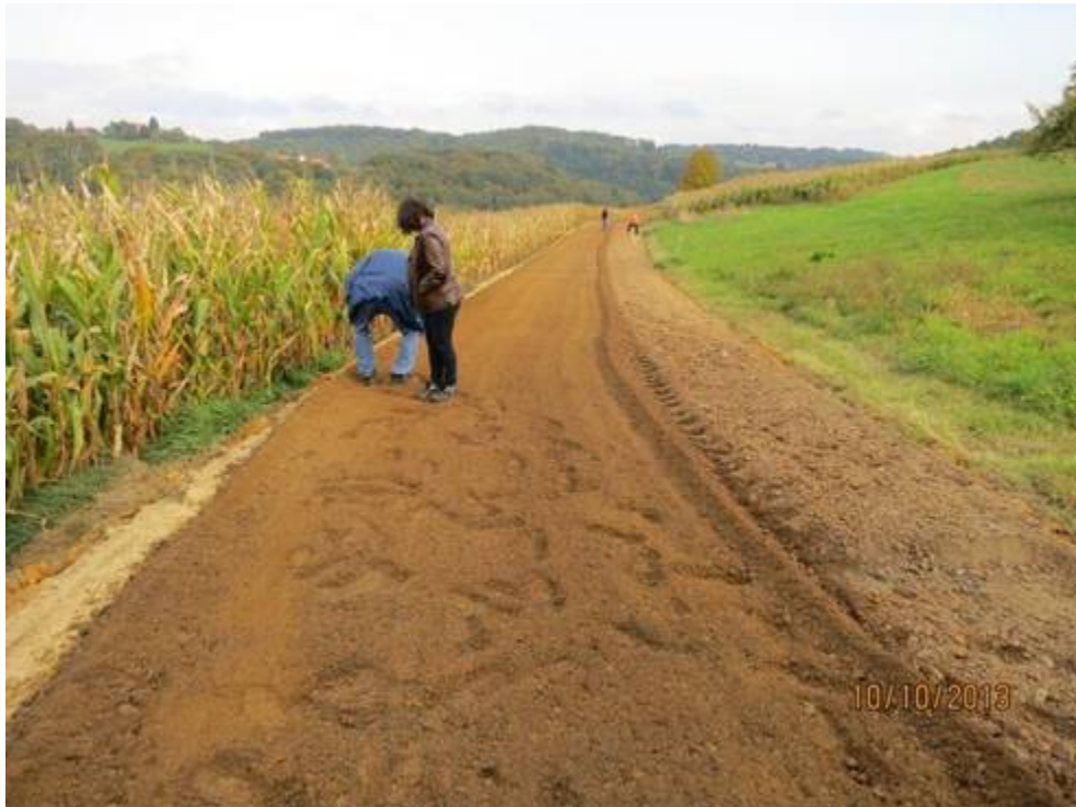
Pulverised road mixed sand-clay-asphalt and gravel underneath asphalt
