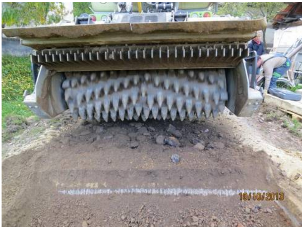
Pulverised road mixed sand-clay-asphalt and gravel underneath asphalt
