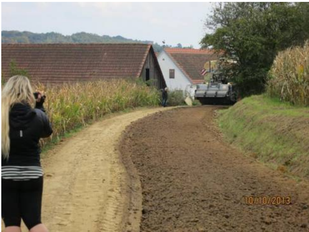
Top photo, view at the west direction – left side pulverize, right side with top sand layer to be pulverize
