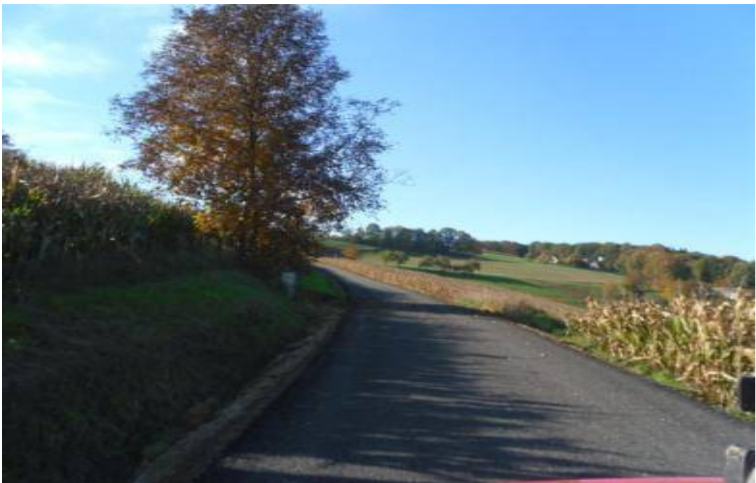
Finished road surface with recycled asphalt
