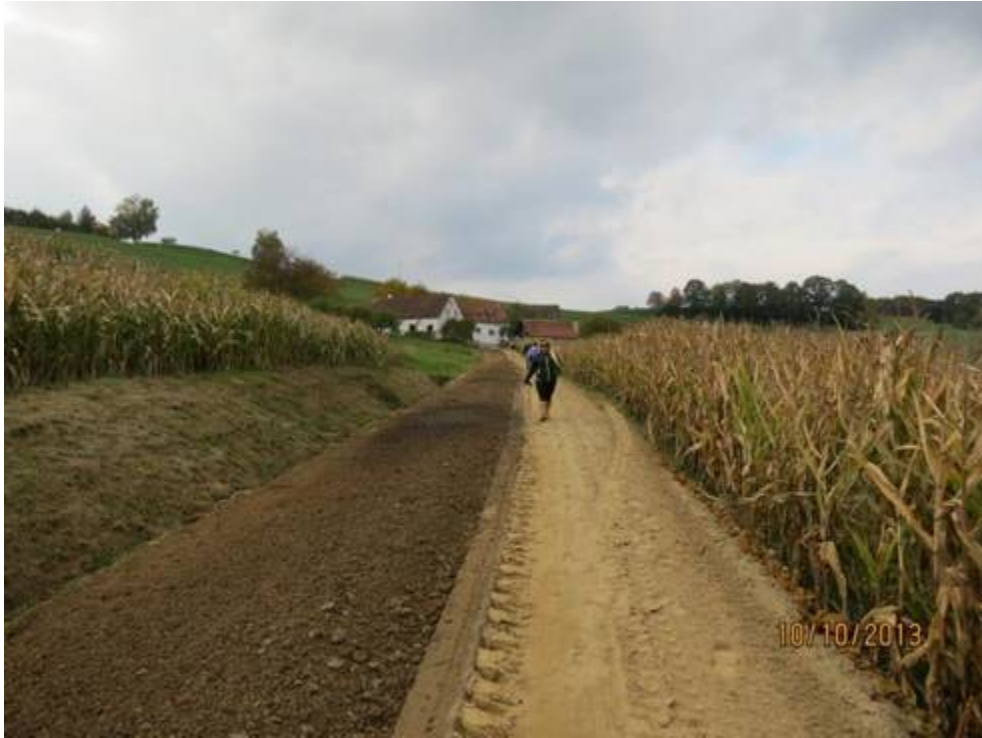
Top photo, view at the west direction – left side pulverize, right side with top sand layer to be pulverize
